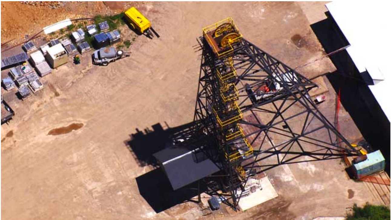
Aerial View of headframe at Morning Star (2010)
