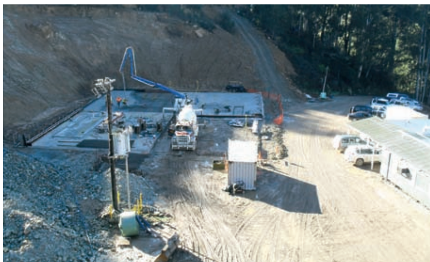
Civil works in preparation for Morning Star's onsite 80ktpa Gravity Mill.
