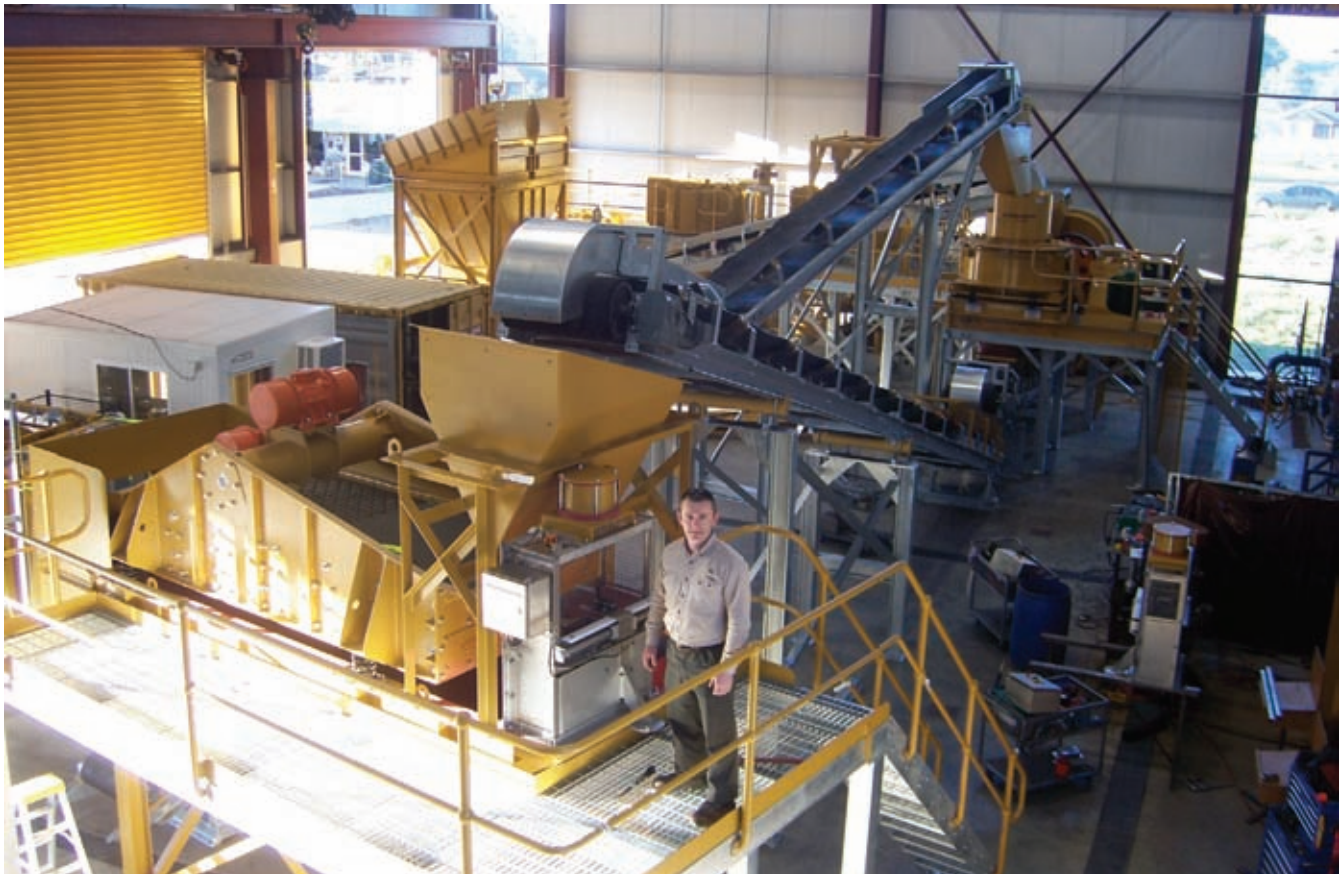
Morning Star Gold is taking delivery of its new 80KTPA gravity gold plant
